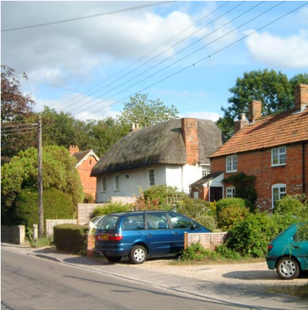
Ashton House was altered in the 19 th century from two cottages but still retains a traditional long straw thatched roof. Alongside are former agricultural workers cottages probably late 19 th century.
