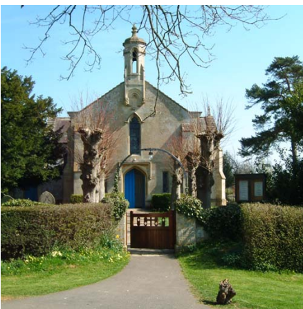
Christ Church was built at the western end of Worton to make it more accessible to the residents of Marston. The secluded location amongst the trees creates a quiet oasis in contrast to the main road. There are open views to the south down to the brook and beyond.
