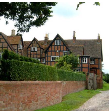
The timber frame, brick and clay tile construction of The Grange is of particular interest as it covers both the 17 th and 19 th centuries. The technique of extending a timber frame building in matching style was popular in the Victorian period.
