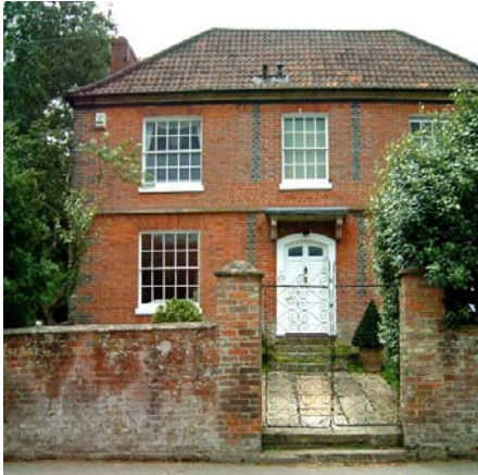
18 th century buildings such as Cambria House are notable for the use of high quality brickwork. Here construction is in Flemish bond and together with double hung small pane sash windows and panelled front door provides a good example of the period.
