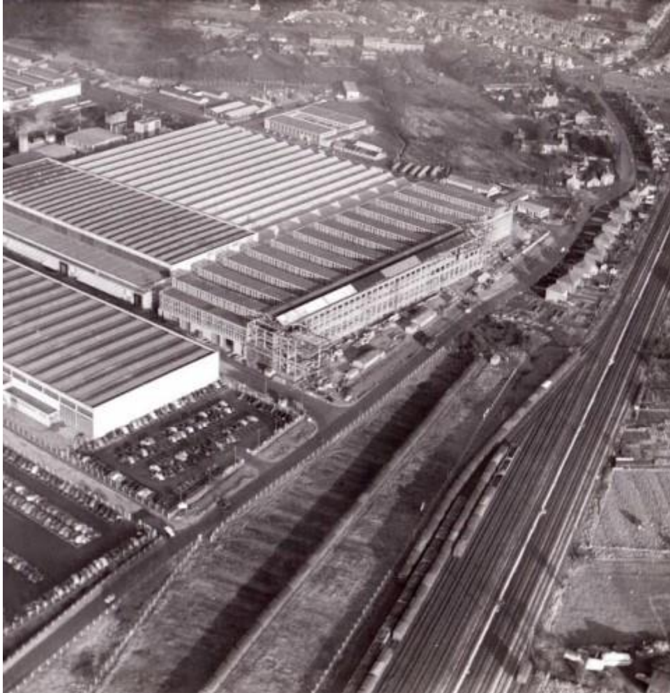
Pressed Steel Plant, Stratton St. Margaret c1960
