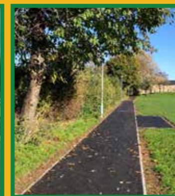
Footpath Refurbishment at Meadowcroft:
