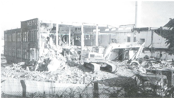
Y Plant being Demolished 1995.
