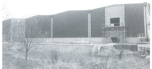
D Plant nearing Completion 1989.
