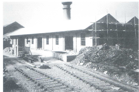
New Warehouse being built alongside the Factory Railway Siding 1950.
