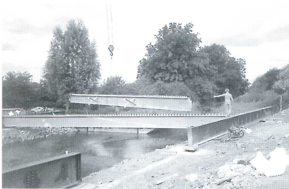
Steel & Concrete Platform being constructed across the Millstream 1987.
