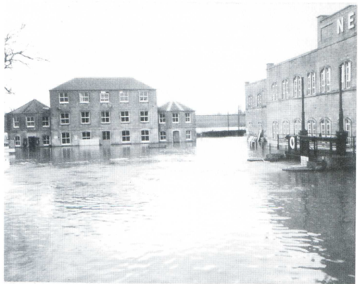
Factory Floods 1960's.
