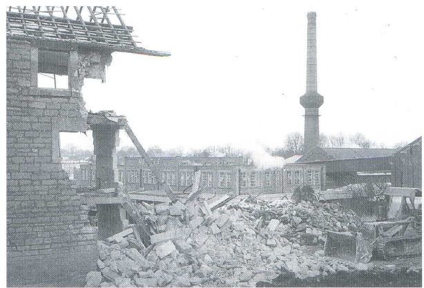
The Rank of old Weaver's Cottages being Demolished 1966.
