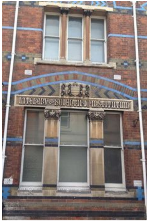
Typical Institution Building
