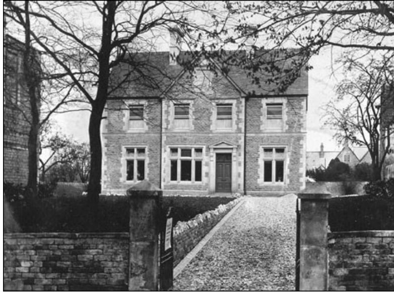
Melksham Cottage Hospital
