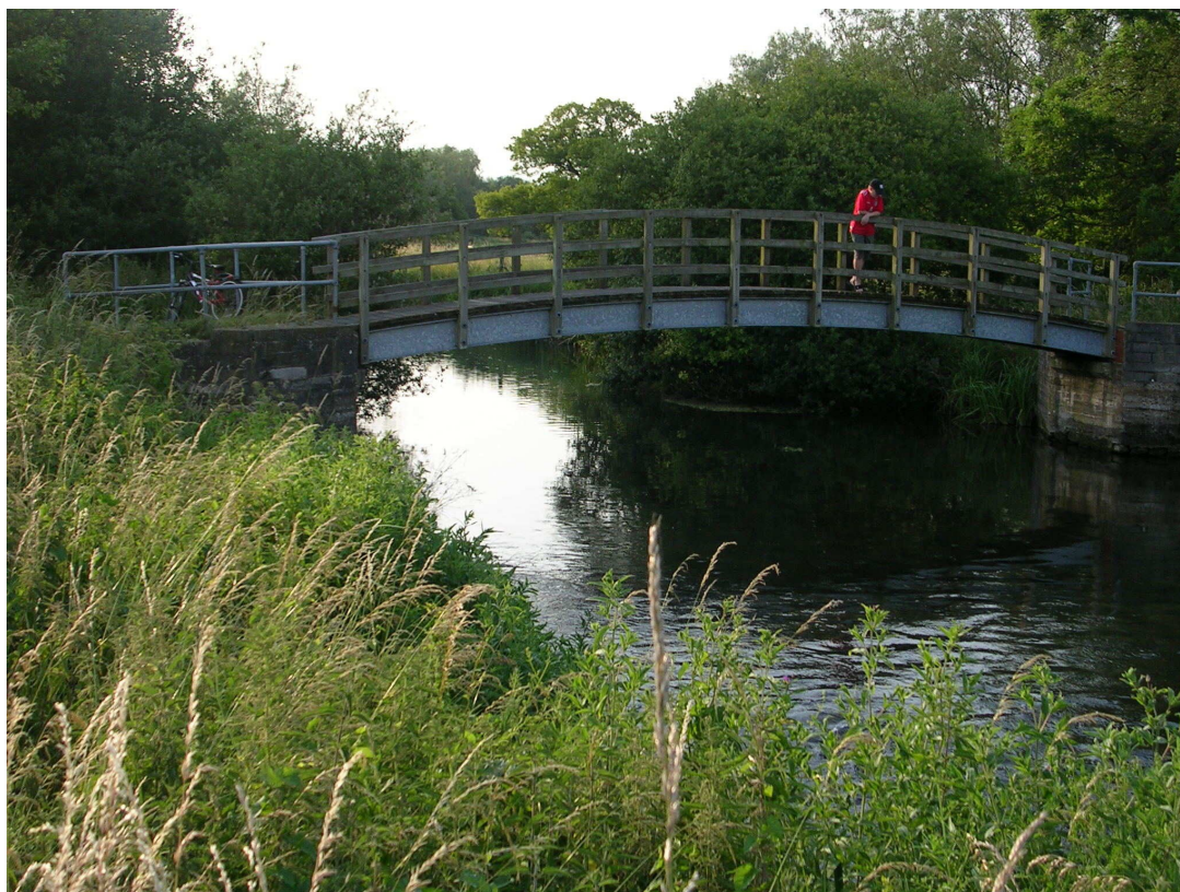
Bonham's Bridge, South Newton c2000
