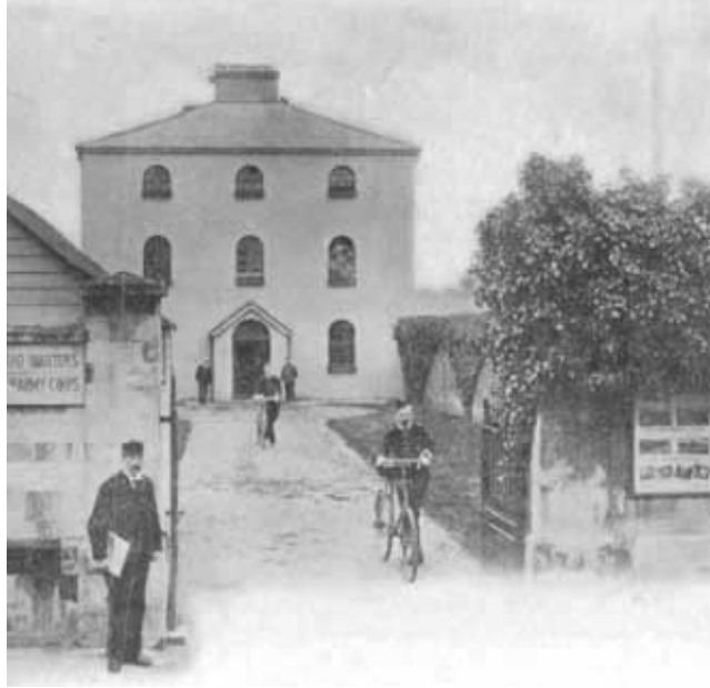
Radnor House, The former Fisherton Gaol
