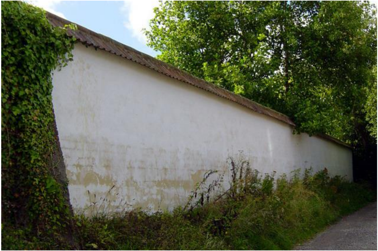
Durrington - Listed Buildings - Wall along Driveway to north of Collins Farmhouse
