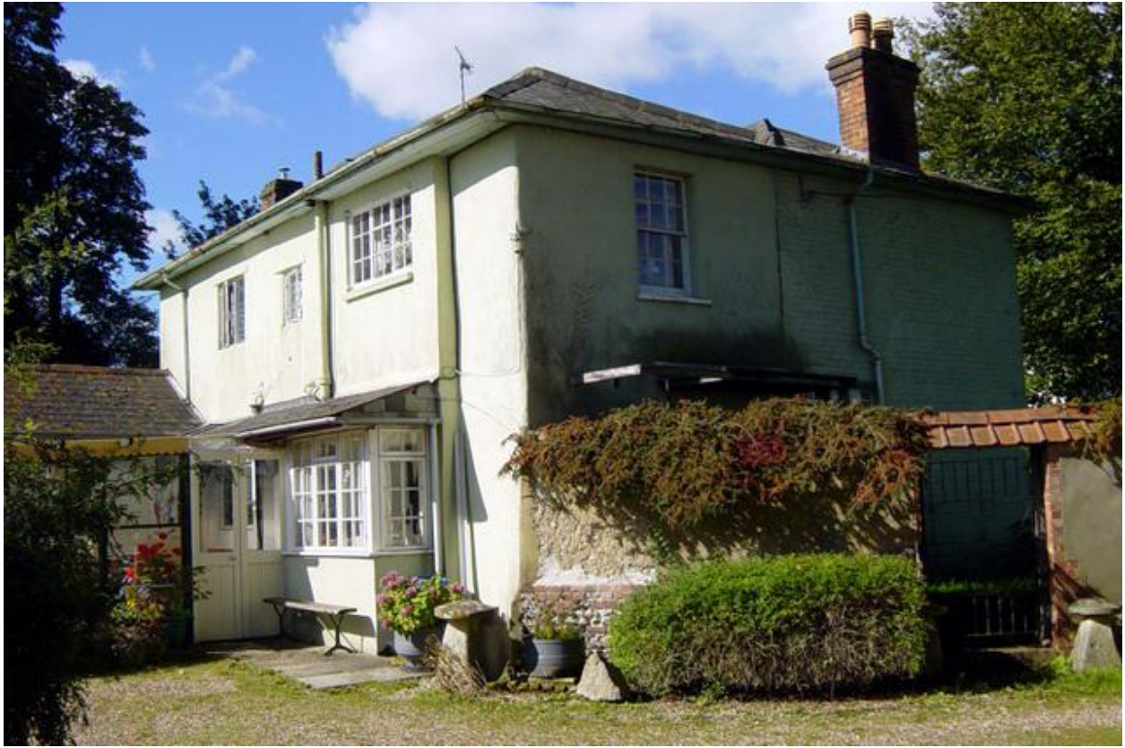
Durrington - Listed Buildings - Church Farmhouse (Photo courtesy of Dave Healing)
