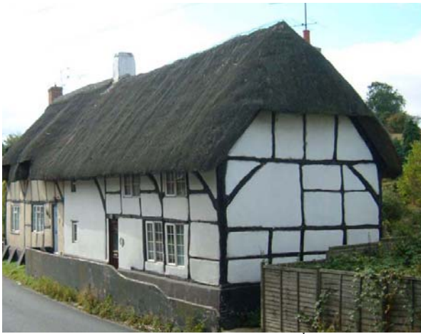
Timber framed cottages of the 17 th century. The original infilling would have been of wattle and daub. The thatched roof is of combed wheat reed.
