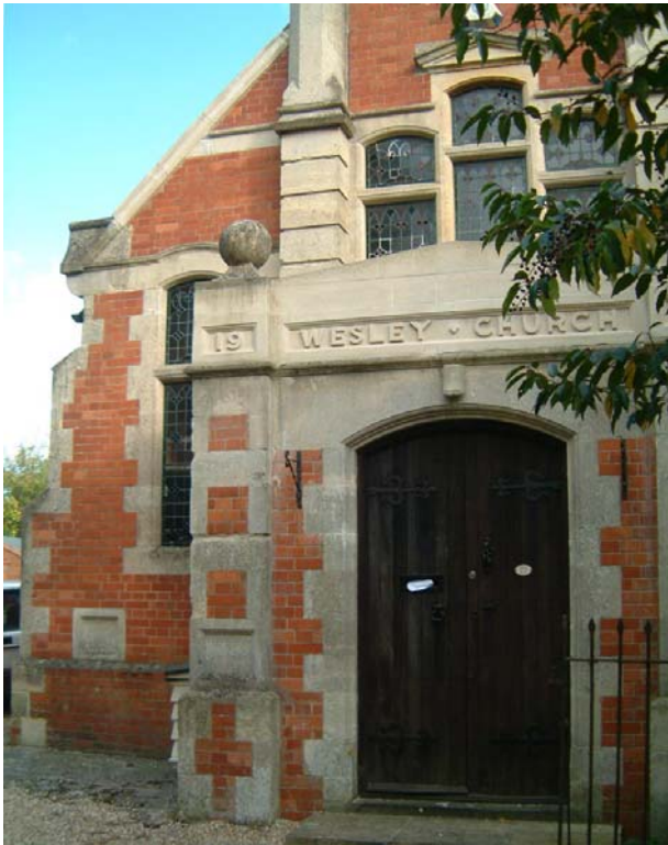
Chapel Lane. The former Methodist Chapel of 1914
