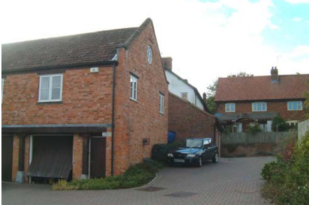
A former granary in Parsonage farmyard was extended and converted to a house and garages. The pair of cottages facing the street front are part of the same 1998 residential redevelopment.
