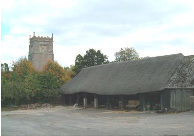
The cart shed at Manor Farm
