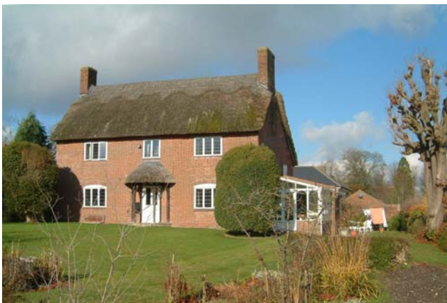
Chapel Lane. Jasmine Cottage of 1777 with a thatched roof of water reed.
