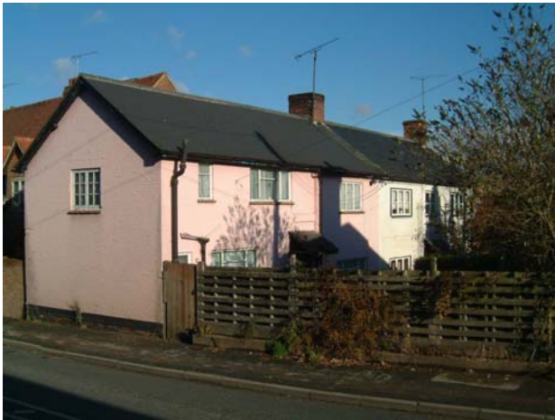
No.s 59 and 60 The Street Rebuilt 1934
