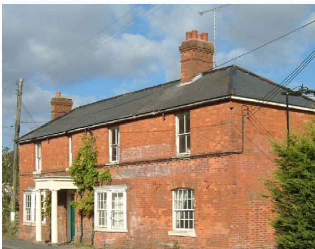
The former Windmill Inn. A hipped Welsh slate roof to a mid 19 th century house. Chimney stacks have single medial band course, three top and a single coggled corbel courses. The nearer stack has four flues each with a matching terracotta pot.
