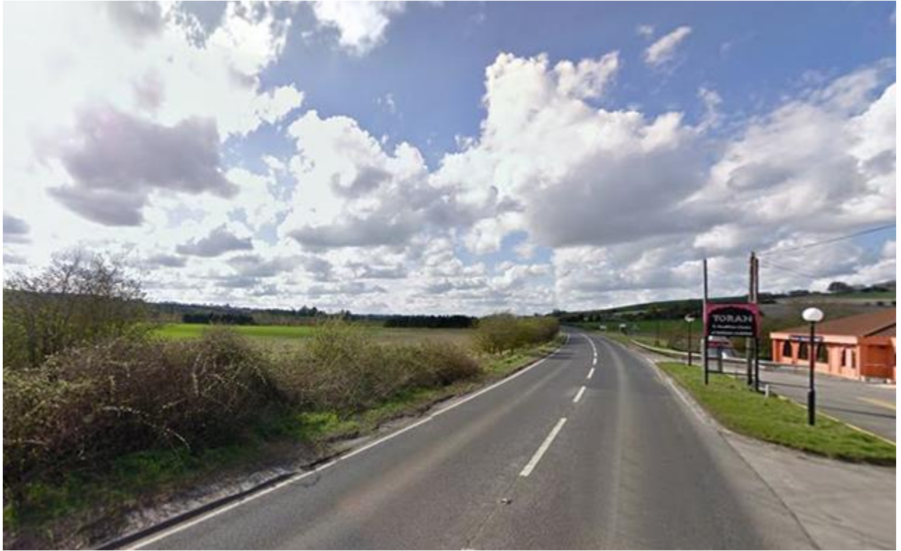
Boundary Post is located on left hand side of A36
