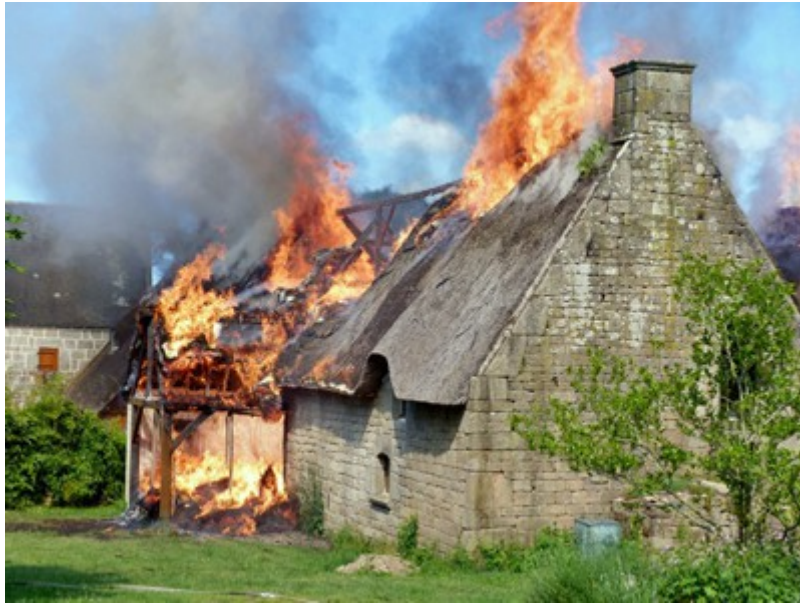
Typical thatched roof cottage fire
