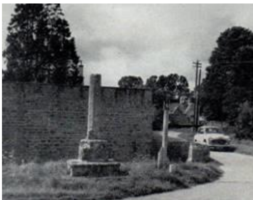
The second cross, the river runs between the wall and the cross
